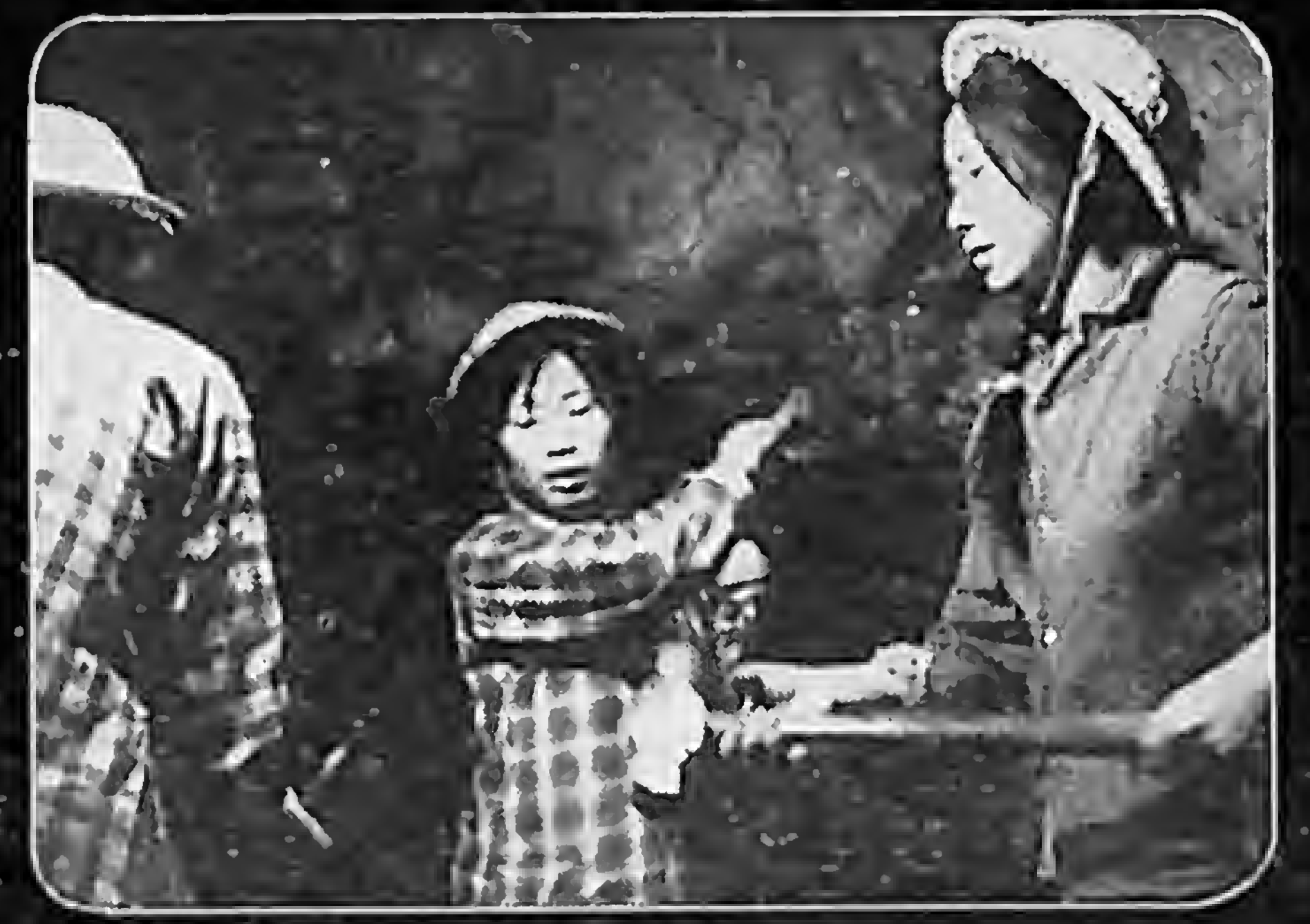
The "Iron Girls" drill team working in the tunnel.
